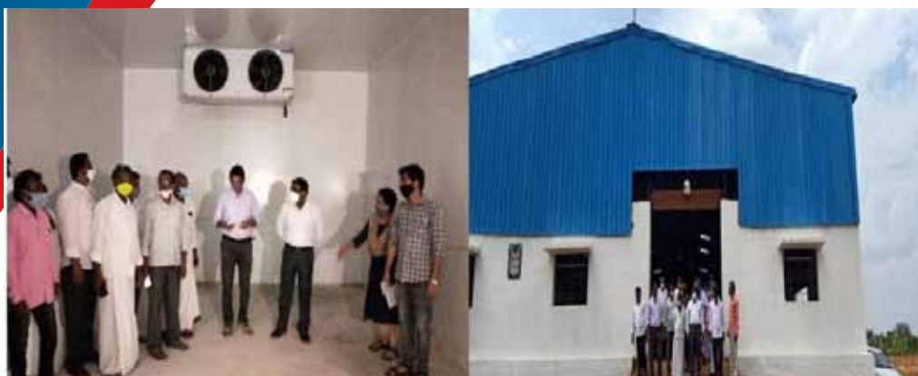
Establishment of Ripening Chamber and Functional Infrastructure under Post Harvest Management by M/s. Annamaiah Raithu MAC Society Ltd., Konduruvaripalem, (V), Piler (M), Chittoor (D), A.P.
